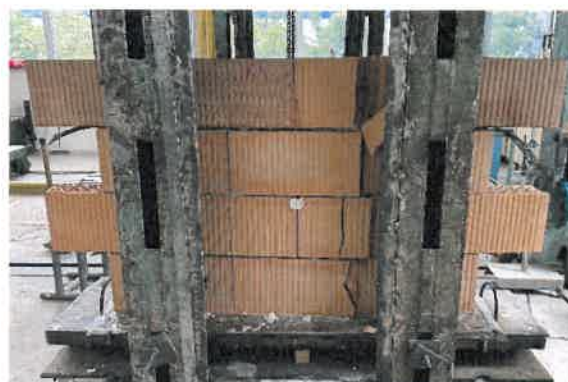
Figure 13 - Failure mode – OK 5
