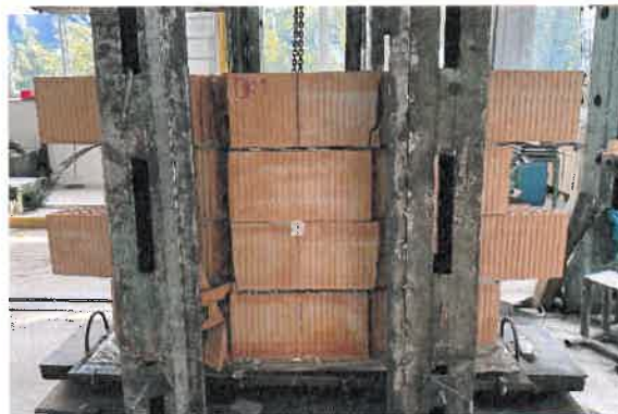
Figure 9 - Failure mode – OK 1
