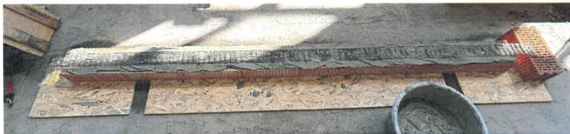
Figure 12 - Assembly of masonry lintel
