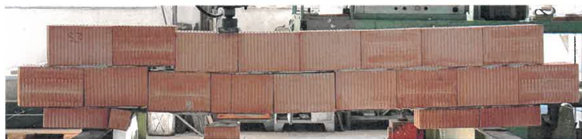
Figure 8 - Failure mode – S3
