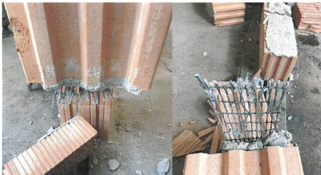
Figure 23 - Detail of torn reinforcement – F 4
