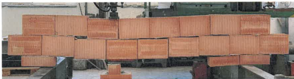
Figure 6 - Failure mode – S2
